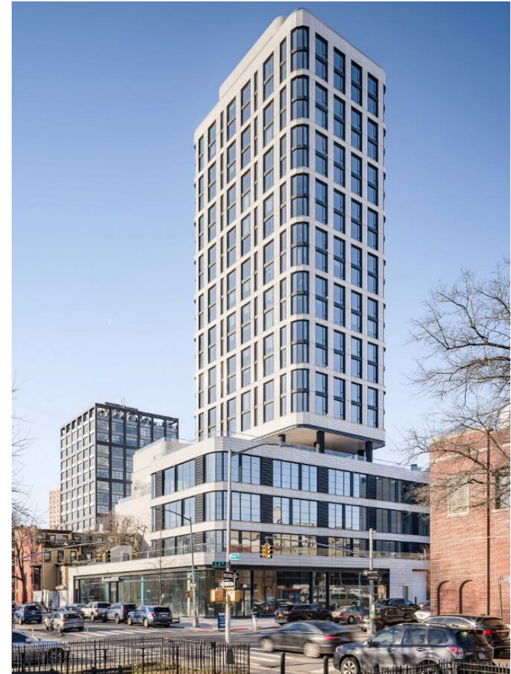
The Dime, Brooklyn: A four story podium provides common open space above and activation on the street.
